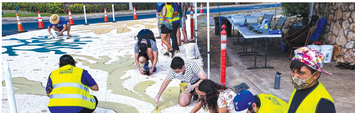
Youth and adults working on a quick-build installation. Source: Ulupono Initiative.
